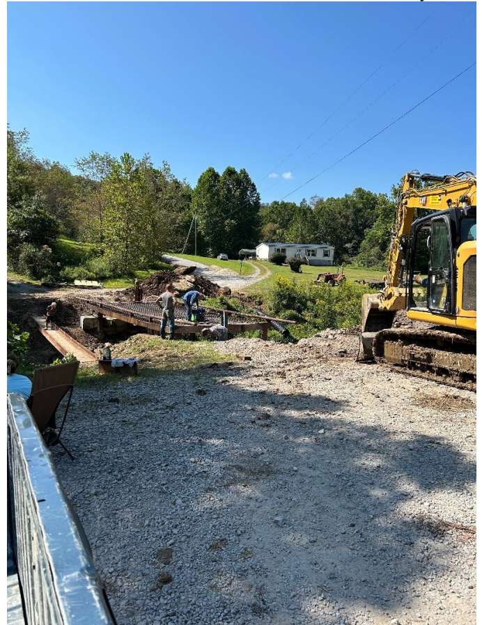
Rebuilding the bridge
